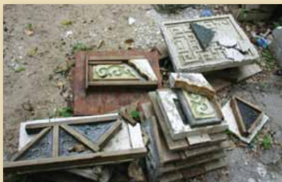
Casting replacement feature tiles on site (King Yin Lei 景賢里)
