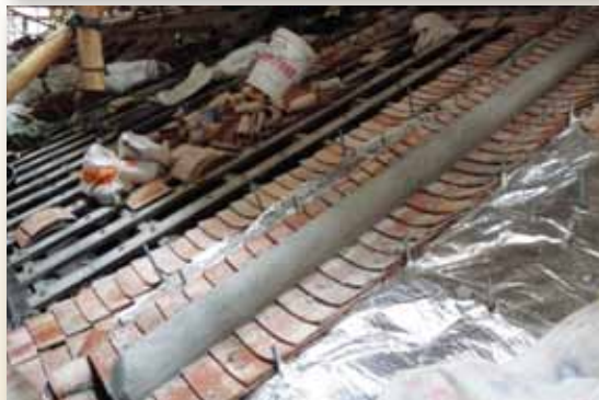
Steel-members reinforced roof structure with matching cover-tiles. (Comix Homebase 動漫基地)
